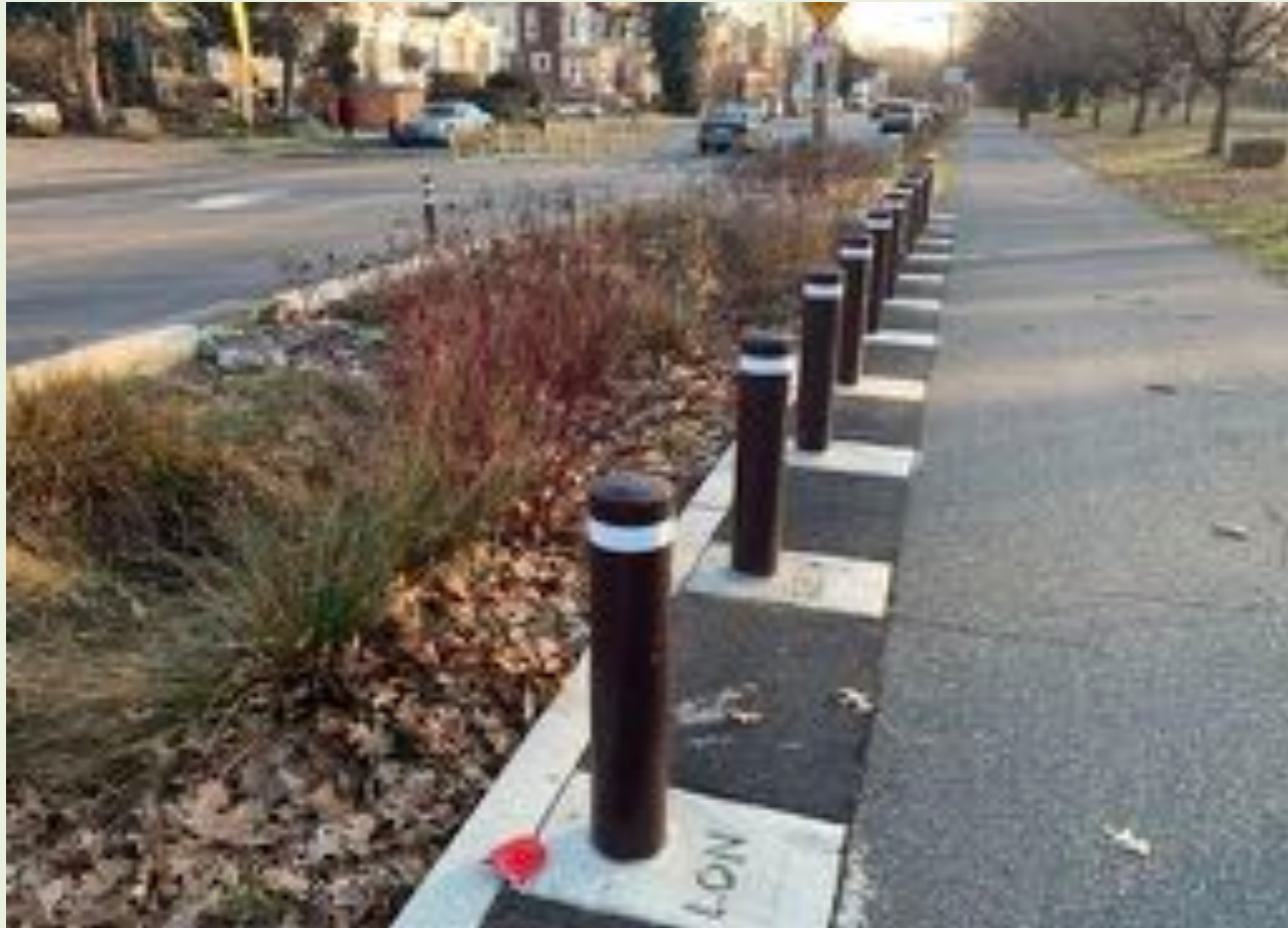
GREEN STORMWATER INFRASTRUCTURE ALONG COBBS CREEK PARKWAY
