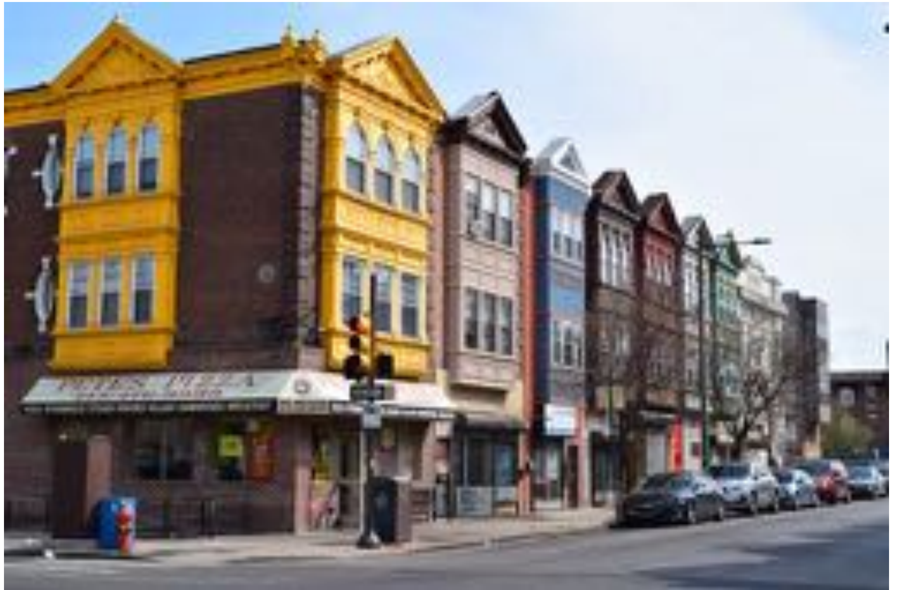
60th Street Facades After Storefront Improvement Program
